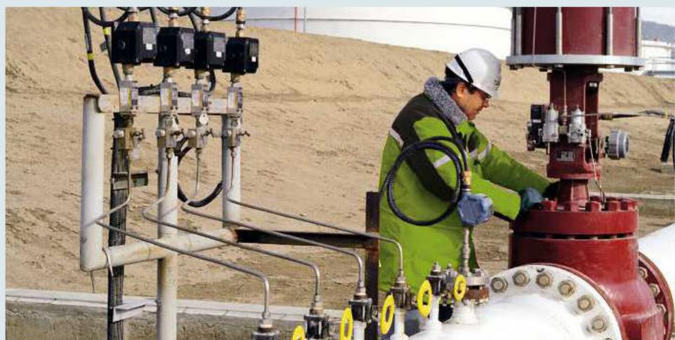
Measurement station sensors on a pipeline
