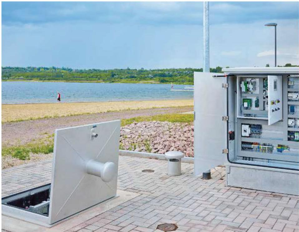
Remote control technology for distributed wastewater pumping stations
